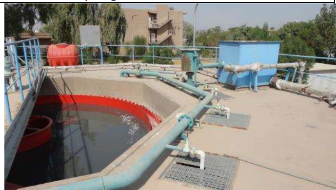
Waste Water Installation
